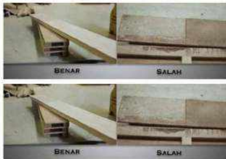
Gambar II.413 Kualitas Cetakan/ Bekisting
