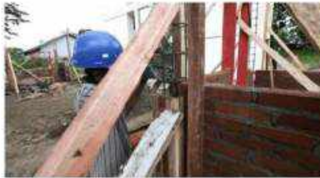
Gambar II.415 Proses Pengecoran Kolom
