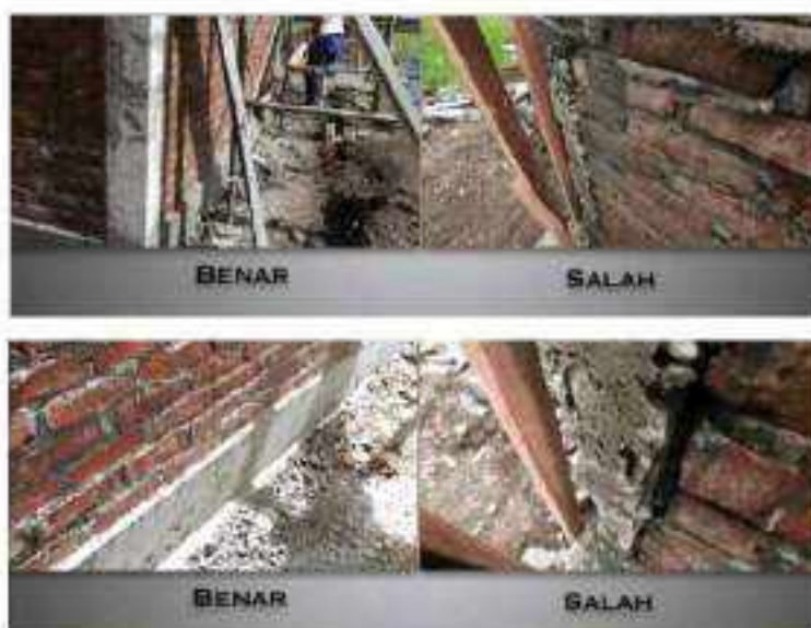
Gambar II.417 Hasil Pengexoran
